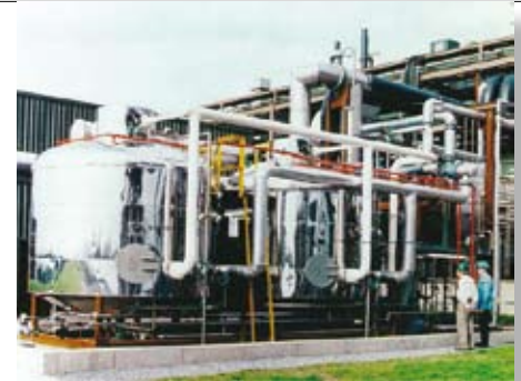
Carbon adsorption system for VOC abatement
